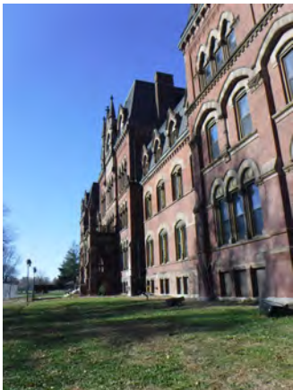
South Facade looking west
