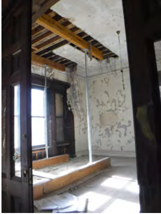
Shoring example on second floor
