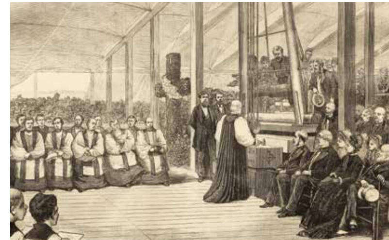
Mrs. Stewart at the laying of the cornerstone at St. Paul's
