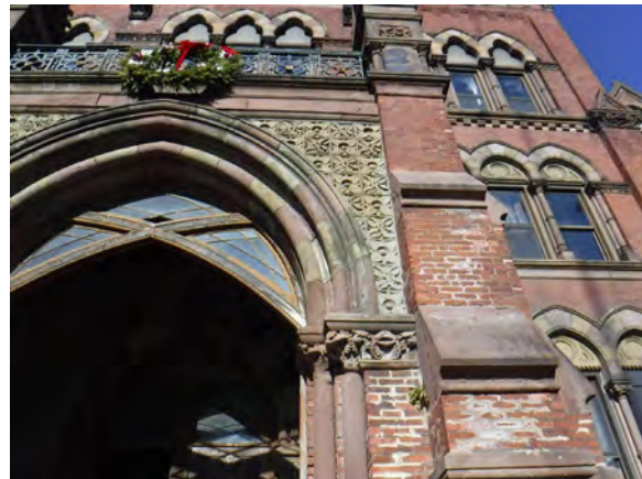
South Facade entry
