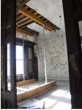
Shoring example on second floor
